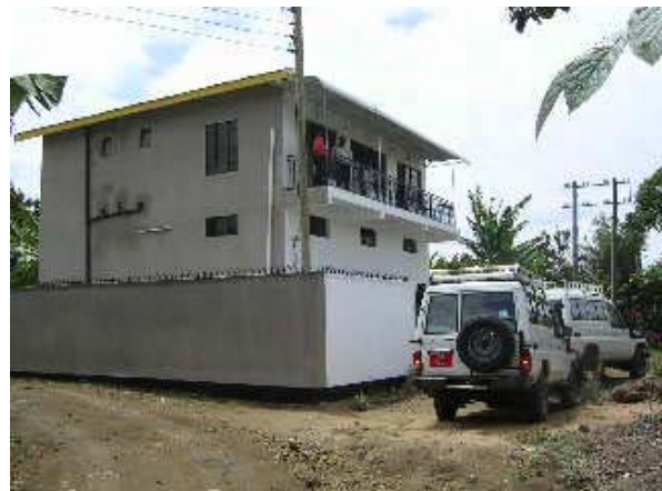
The Transshipment Point (located few kilometres from Arusha Municipality) which will be used by facilities to collect their deliveries from the Prime vendor.
